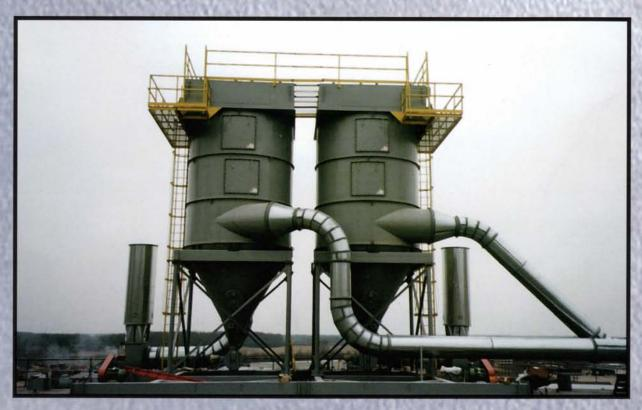
A picture made during the installation of these dual CAR 193-10 units [above] shows them before locating overhead lights or connecting walkway grating.
