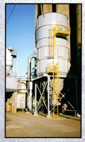
The discharge from a larger 16-ft. diameter baghouse, model 16RA412-10 (facing page, upper right, lower right) is carried by a high-pressure line into a bin for truck load-out. Caught amid its installation, another 16-ft. diameter baghouse (above left) rests on a custom-made steel support far above grade.
