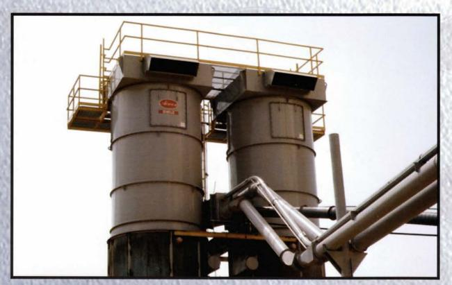
For nuisance dust from the by-product trash tanks below, a couple of CAR 101-10 baghouses [above] were found to be the solution. The total compressed-air requirement for both will not exceed 36 SCFM at 90 to 100 PSIG.
