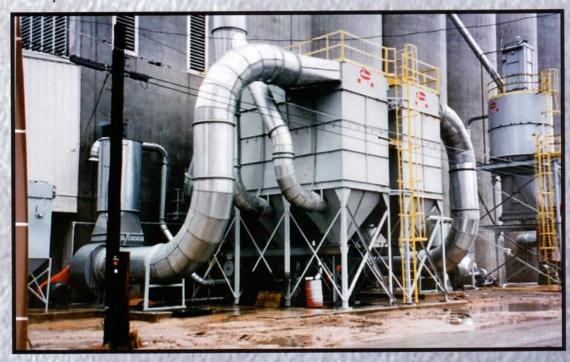
The grinding systems in a feed mill require smaller CAS units [below left & below right], often with screw conveyors and rotary valve (airlocks). Given a certain required filtering area, the CAS has the advantage of compactness over its cousin, the compressed-air round (CAR). On the other hand, the CAR has the advantage of a tangential inlet, which allows for some pre-filtering of the air prior to reaching the filtration bags.
